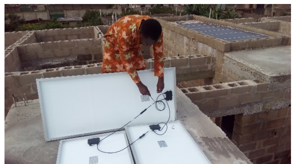
Figure 4: The solar panels being fixed
